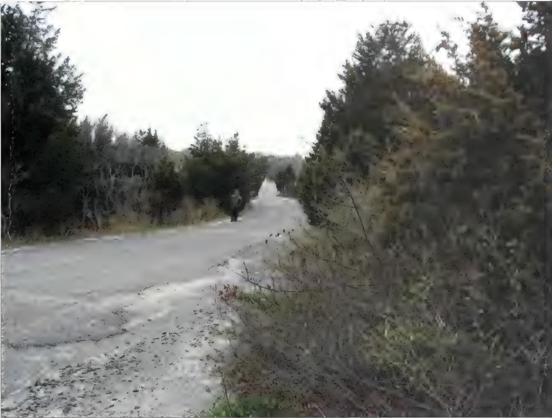
Figure 3.65. View looking west along central access road, NIKE launch site. Heading east from the Ready Barracks, the topography rises along the central access road to the missile magazines (Olmsted Center, April 2008).
